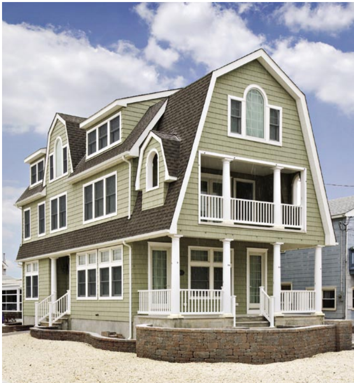
Challenging to build, this 3,000-square-foot Dutch Colonial-style beach house was creatively designed to fit on a very narrow lot with views of the ocean and bay. The exterior is finished in CertainTeed Double 7 Cypress siding with a GAF Timberline Lifetime roof.
